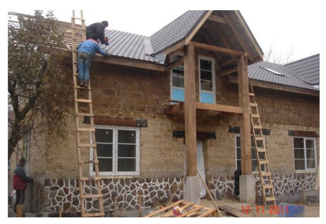
PICTURE 4. Construction of straw brick houses in Kyrgyzstan. Source: construction portal USTA (www.usta.kg)
